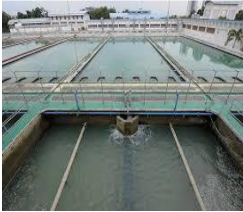
Shut down of water treatment plant due to river pollution
