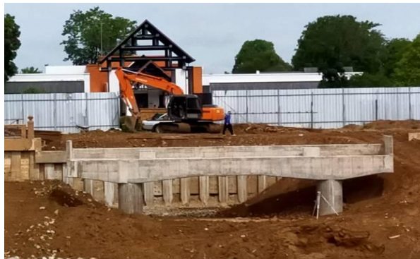
c) Construction of crossbeam
