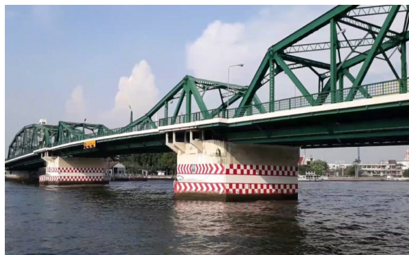
Figure 9 - Pan Fa Lilat Bridge (Re-built)
