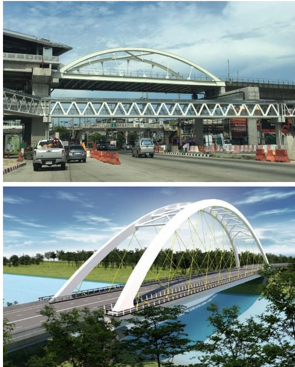
Figure 13 - MRT arch bridge
