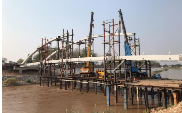
a) Installation of approach span
