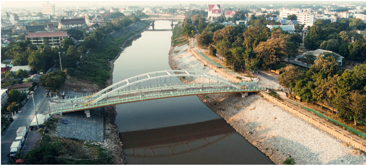
Figure 7 - The bridge when it completed
