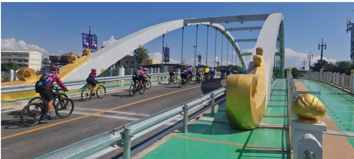
Figure 8 - The bridge as a part of bike trail
