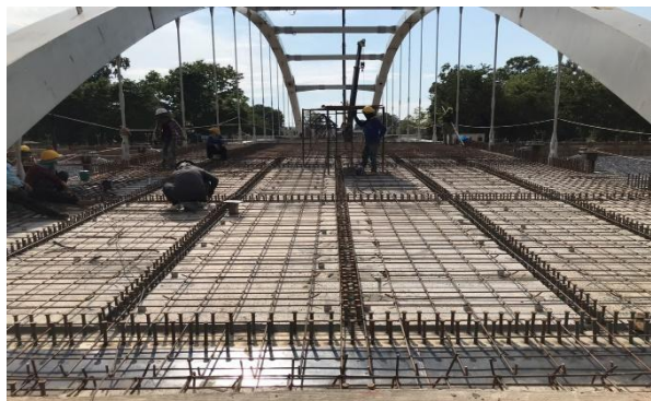
c) Installation of hanger rod
