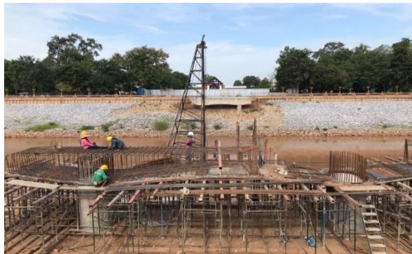
a) Bored hole drilling
