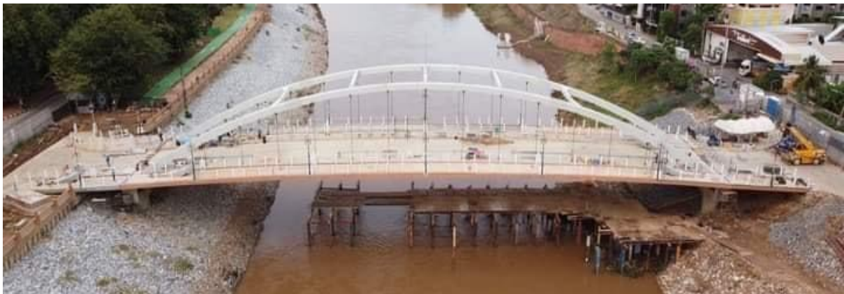
g) Completion of superstructure installation
