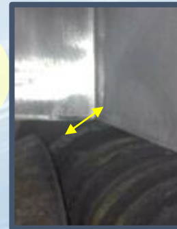
Photo of slab corner defect and associated mold problem
