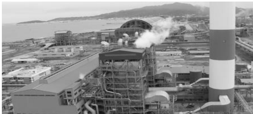
Figure 3.6.2 Bird's eye view of the Steam Power Plant
